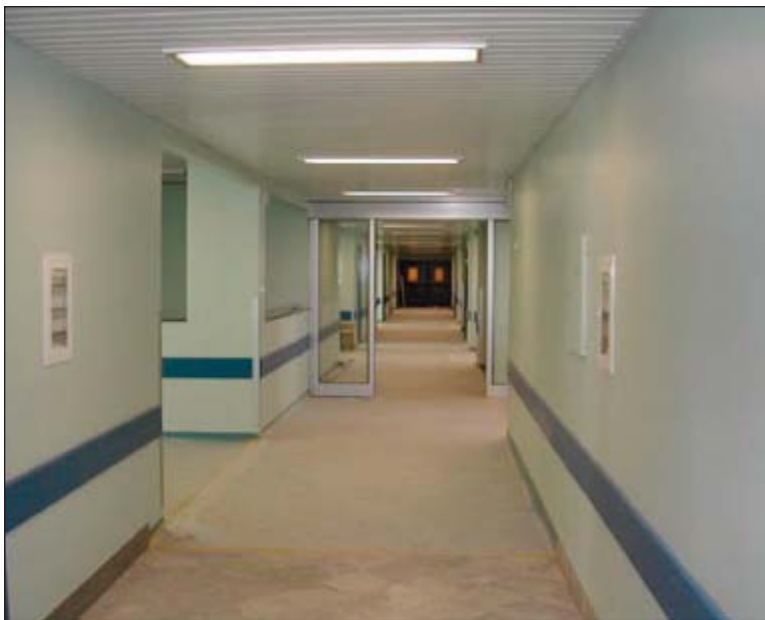
CPHA managed the renovation of the Pristina University Hospital's maternity ward through a CIDA-funded post-conflict reconstruction initiative for the UN-administered province of Kosovo. Before the renovations started, wastewater was leaching through the walls; after the renovations and the application of hospital infection control and housekeeping practices (in partnership with Kingston General Hospital) a hospital ward in excellent condition
