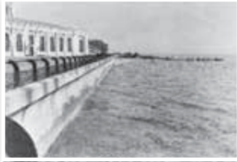
R.C. Harris Purification Plant, view from tunnel shaft, September 2, 1953
